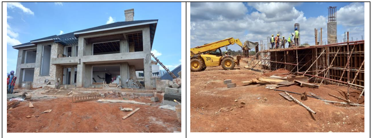
Figure 3: Construction activities taking place in Tatu City phase 1
